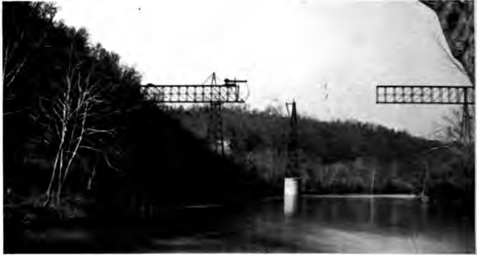
HIGH BRIDGE UNDER CONSTRUCTION. The first cantilever bridge built in America.
